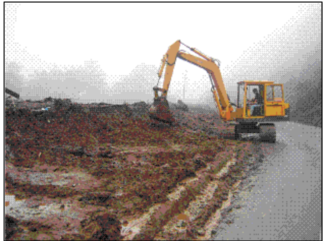
Clearing of mud from the landslides one month after
